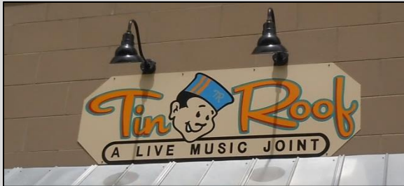
Above: This wall sign utilizes exterior lighting featuring cutoff light fixtures to reduce glare.
