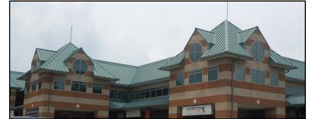
Above: The articulation of this stage set roof breaks up what could be an expressionless façade.
