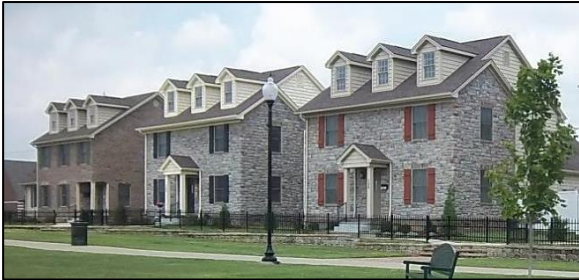
Above: New single-family dwellings should be developed at the same or higher density than currently exists.
