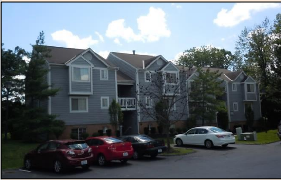
Above: A wide range of architecture is allowed for multi-family buildings to accommodate different styles and densities of development.
