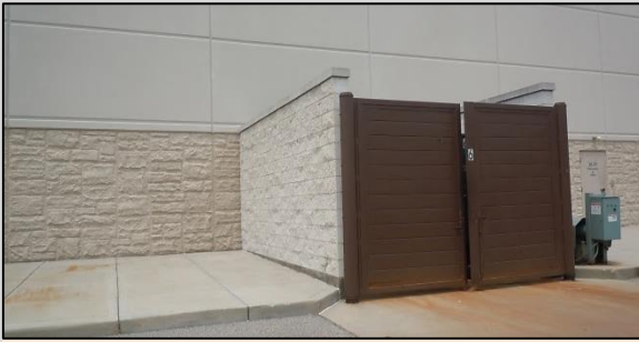
Above: The use of similar building materials and comparable colors integrate a trash enclosure into a building.
