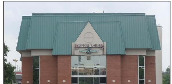
Above: The size and scale of mansard roofs overpower and detract from the character and form of a building or structure.
