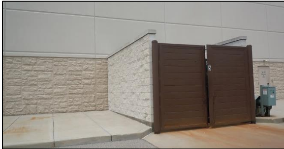
Above: The use of similar building materials and Comparable colors integrate a trash enclosure into a building.
