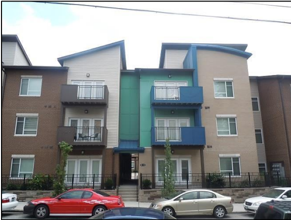
Above: Multi-family buildings can range from moderate to very high density.
